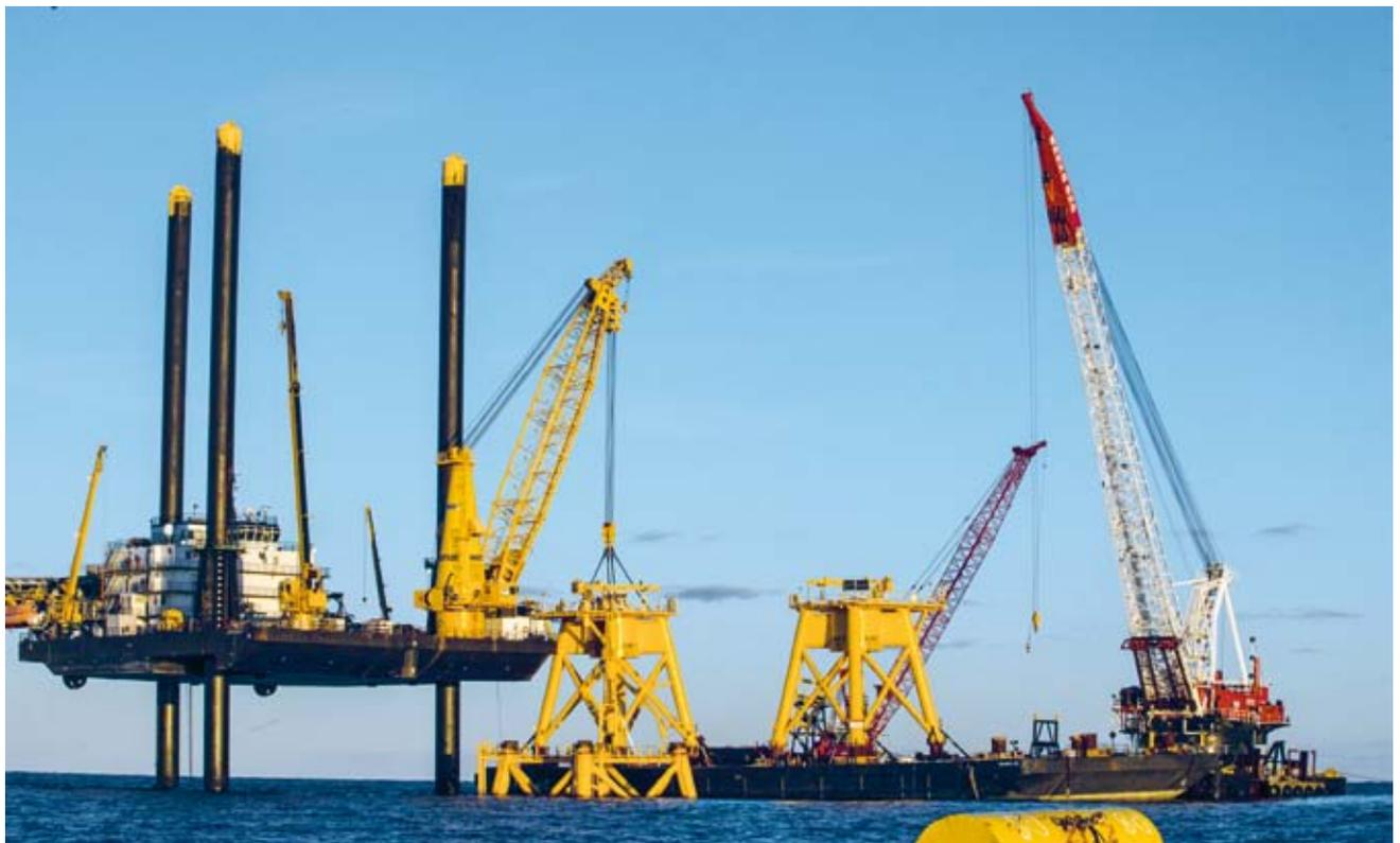
The foundations for the turbines of Block Island Wind Farm are being put in place. We insure construction and start-up delay risks of this project, the first-ever offshore wind farm in the US.
