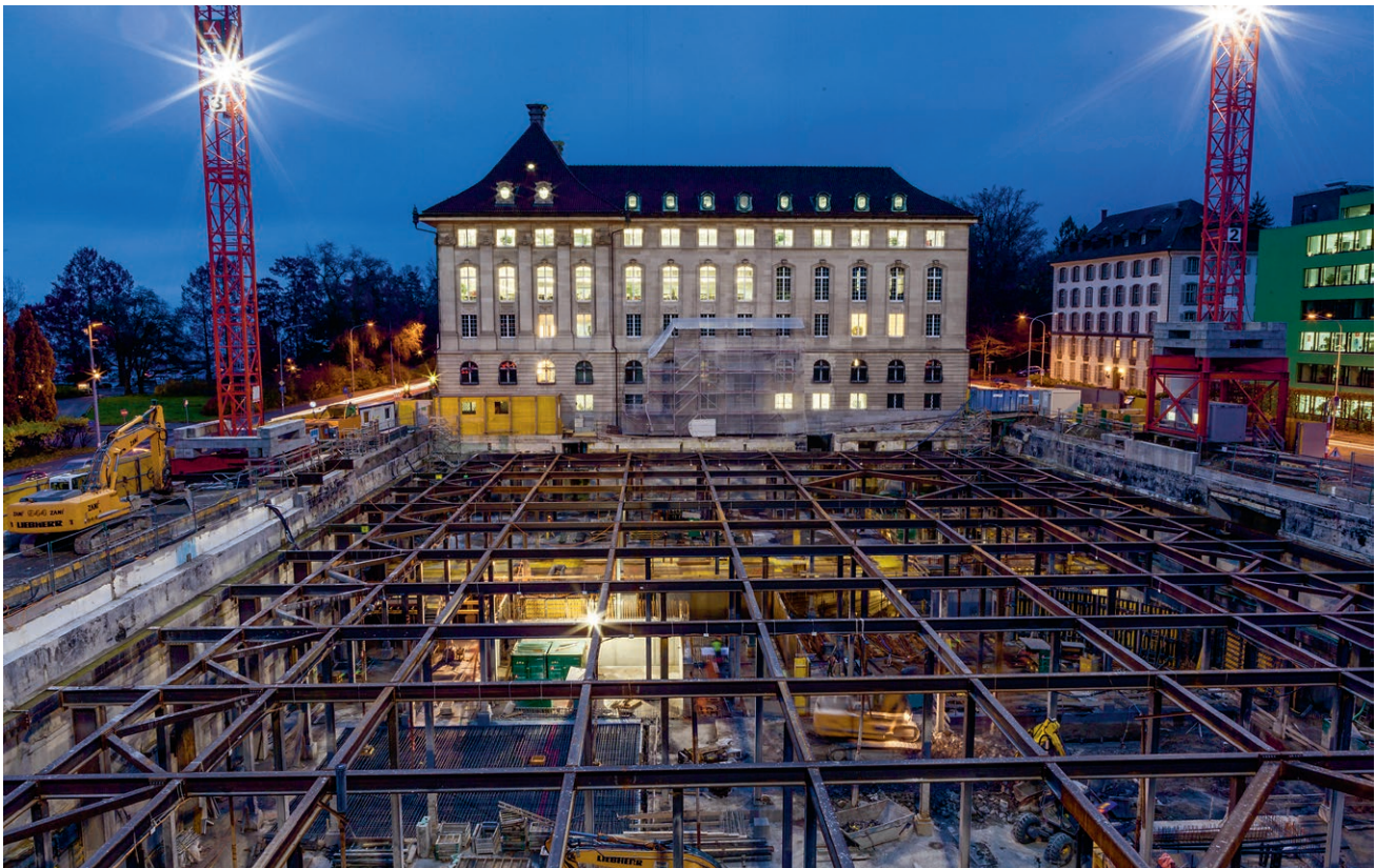
The groundwork is being laid for Swiss Re Next, our new headquarter building that will set a leading example of sustainable construction. The “strut platform” shown in the picture was erected to support and preserve the existing excavation enclosure made of 60 cm thick reinforced concrete. Originally constructed in the 1960s for the previous Neubau building, it is still in superb condition today.
